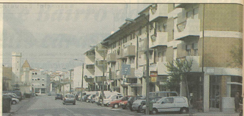
Rua José Luciano de Castro, artéria principal de Esgueira
